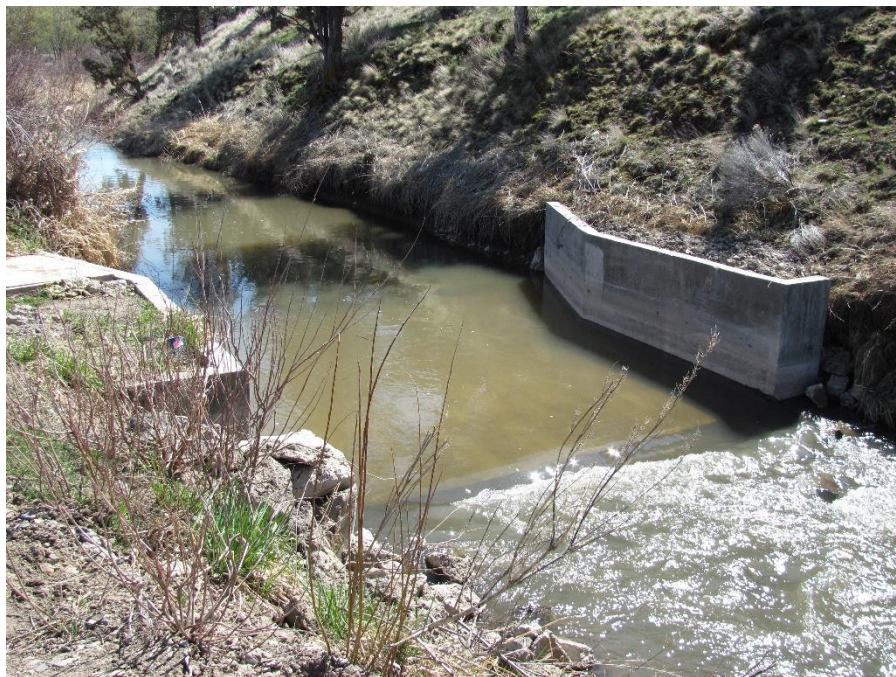
Figure 1. Peoples Irrigation Diversion Canal Measurement Flume (Photo provided by OWRD).
